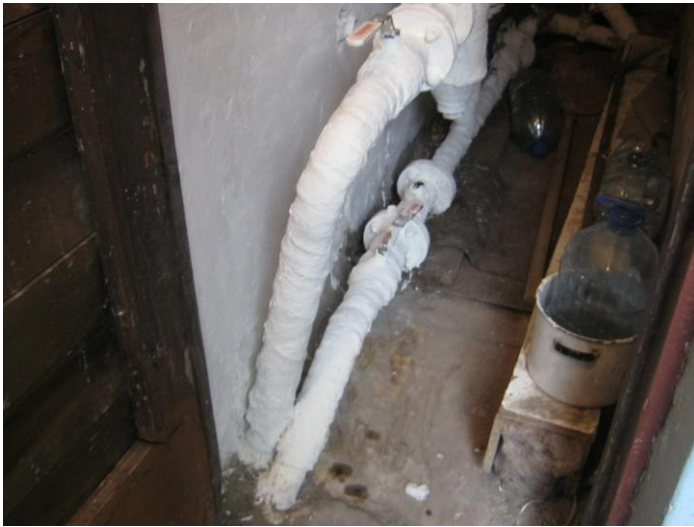
Photo and thermogram. Pipes treated with Isollat liquid insulation
