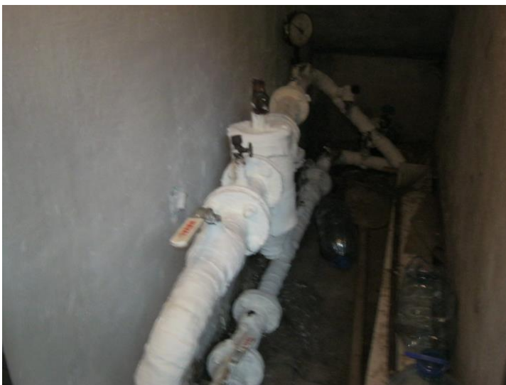
Photo and thermogram. Pipes treated with Isollat liquid insulation
